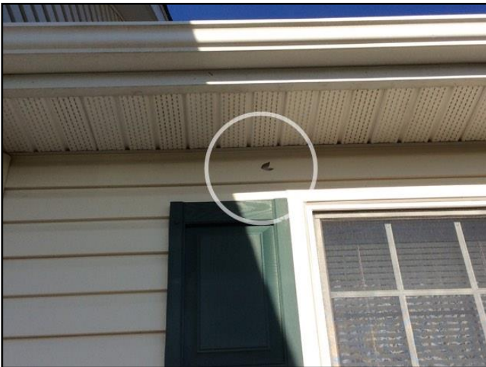
3. Mechanical damage
