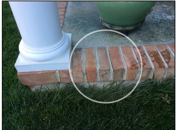
8. Typical minor cracks
